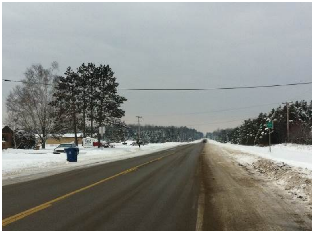
M-55 at the east side of the township
